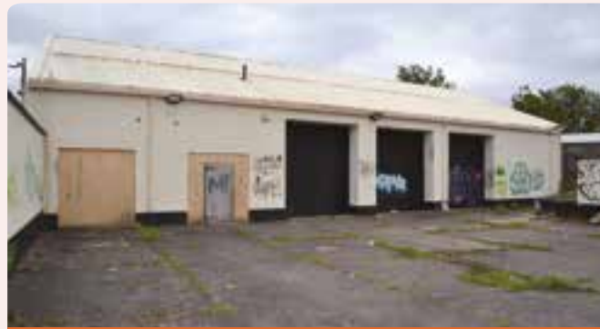
Exterior prior to renovation
