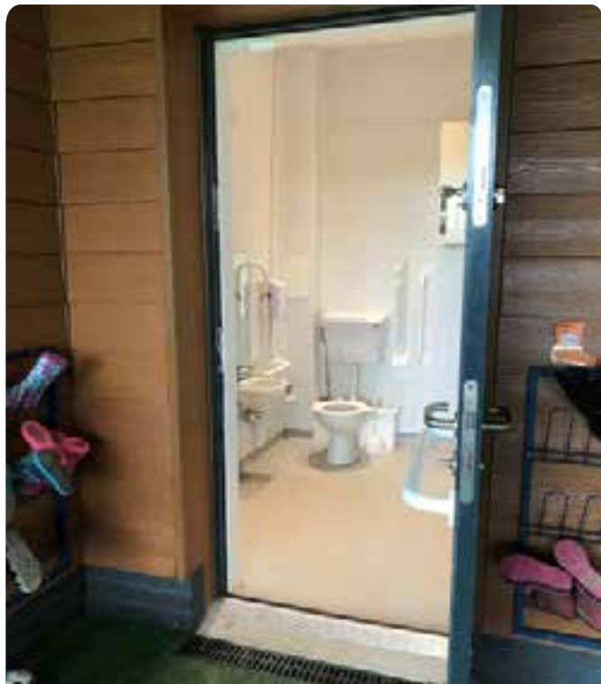
Children at Kelvinside Academy Nursery have a toilet they can access easily when outdoors
