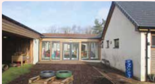
Corridor linking both buildings
