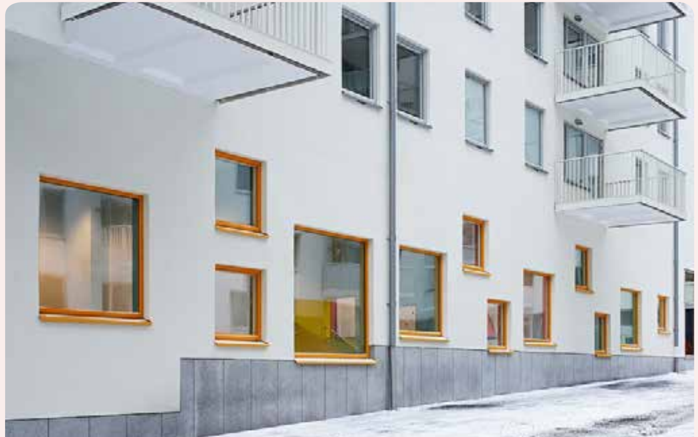
Setting provided from ground floor of residential building, Rotstein Arkitekter
