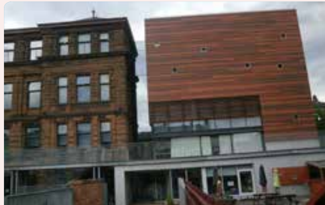
Extension added to listed building. Setting provided from ground floor
