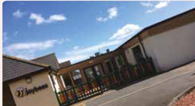
Original accommodation links to renovated workshop
