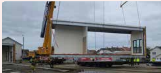
Lynburn Primary School Nursery, Dunfermline, Fife - construction
